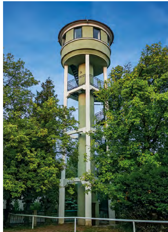
074 Water tower converted into a viewing tower. View from the southeast. Photographer: Magdaléna Straková.
