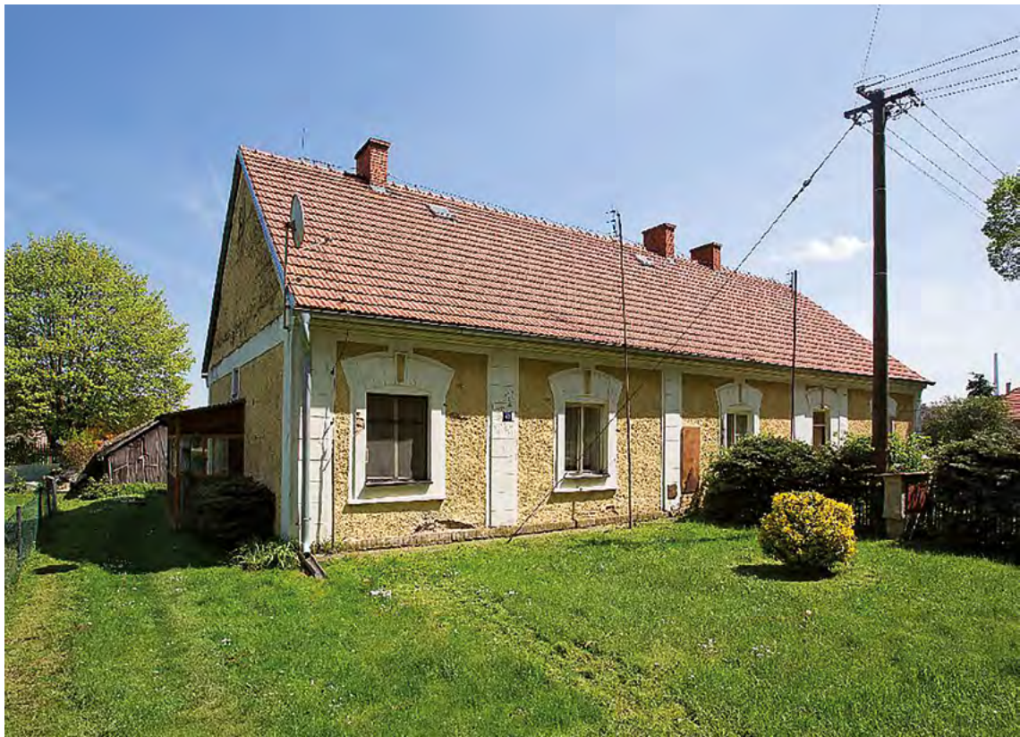
089 Former poorhouse at Selmice built in 1898 to celebrate 50 years of Emperor Franz Joseph I on the throne. Now the building is used for temporary accommodation of employees. Photographer: Jiří Podrazil.
