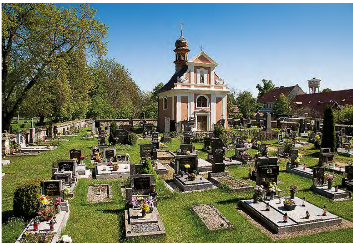
068 Graveyard Chapel of the Exaltation of the Holy Cross at the Kladruby nad Labem farmstead. View from the south. Photographer: Jiří Podrazil.
