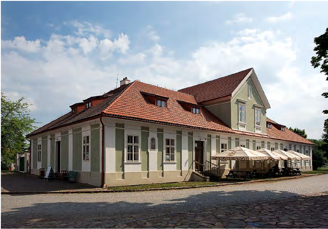
085 Former Imperial Inn at Kladruby nad Labem converted into the visitors centre (it includes a multifunctional conference room, information centre and restaurant for visitors). Photographer: Jiří Podrazil.
