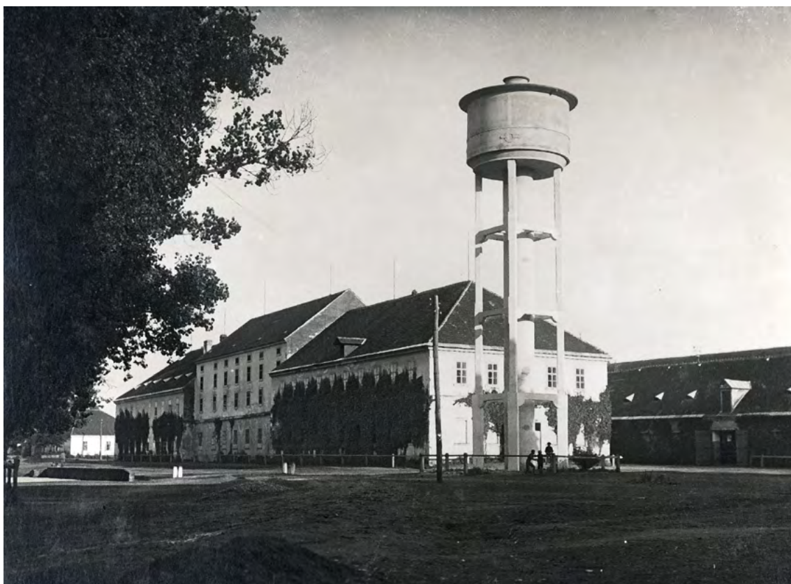
012 View of the stable buildings at the Kladruby nad Labem farmstead with a new water tower. View from the northwest. Photograph from the 1930s. National Stud Farm at Kladruby nad Labem, s.p.o. Archive.
