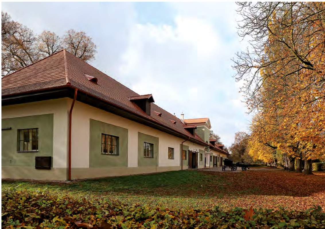
071 South wing of the building ensemble at the Kladruby nad Labem farmstead (Tack Room, Coach House and the Řečanská Gate). View from the northeast. Photographer: Jiří Podrazil.
