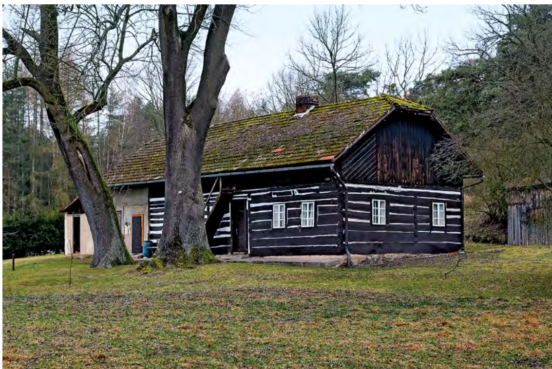
088 Game keeper's lodge in the central part of the Nominated Property situated between the production forest and grazing fields at Na Sklepích. Photographer: Jiří Podrazil.
