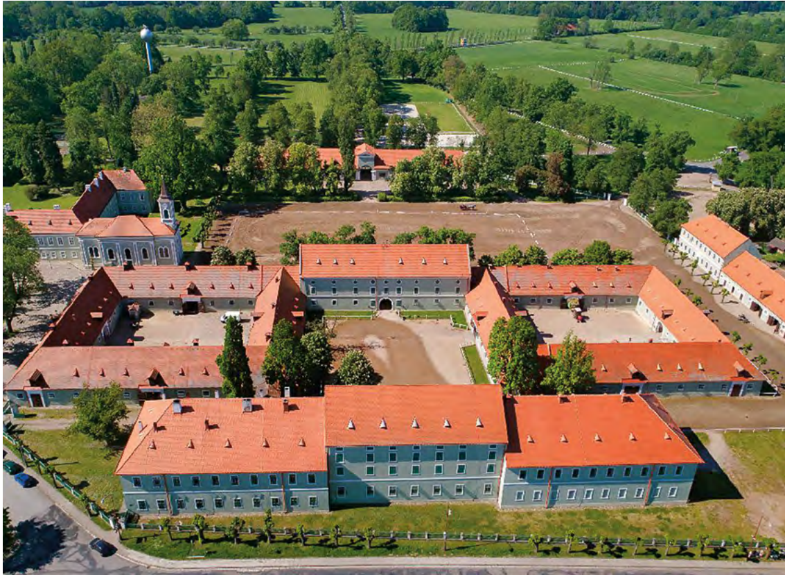
054 Kladruby nad Labem farmstead with St Wenceslas and Leopold church joined to the Manor House and the Řečanská Avenue in the background. It starts at the farmstead south gate. View from the south-east. Photographer: Jiří Podrazil.
