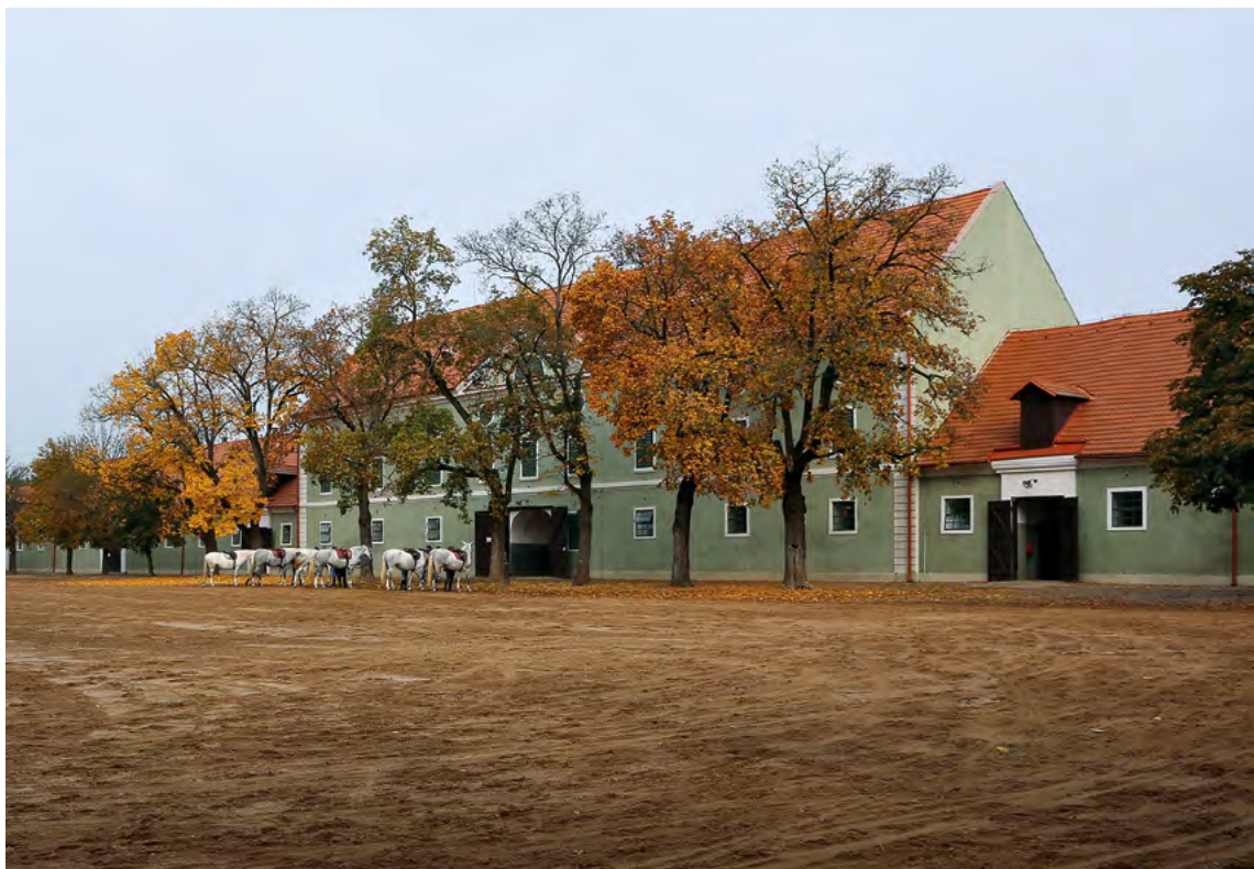
060 Stables at the Kladruby nad Labem farmstead. View from the southeast. Photographer: Jiří Podrazil.
