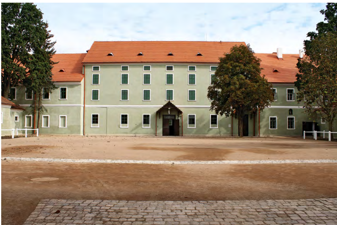
058 Stable of studs. View from the southwest from the inner court. Photographer: Šárka Veinhauerová.
